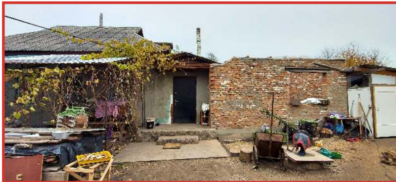
The kids carried used bricks from the village to help build this small room. There is no window. It needs to be completed.
